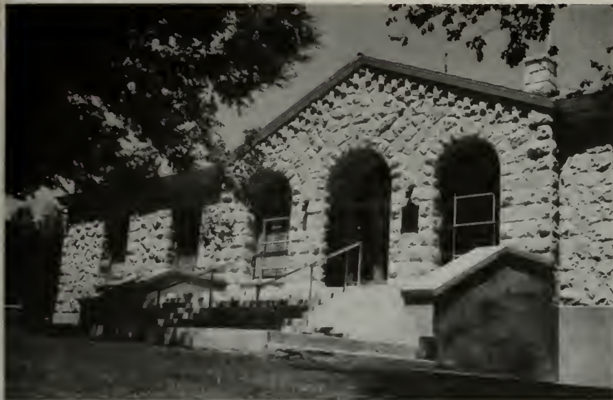
Photo 33. Alpine County Courthouse in Markleeville. This building was constructed in 1928 of blocks of rhyolite tuff that were obtained from Silver Mountain City. Camera facing east.
