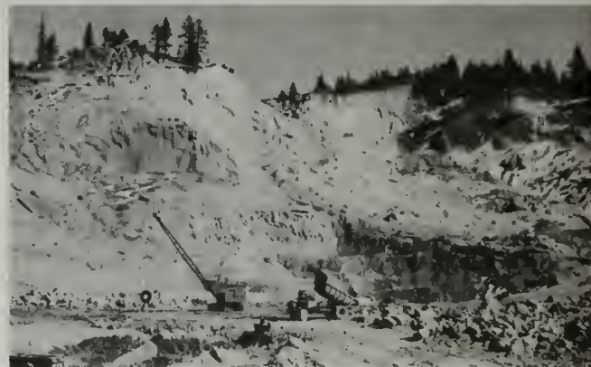
Photo 35. Mining operations at the Leviathan sulfur mine in 1962 showing drop ball used for secondary breaking of large fragments. Camera facing east. Photo by Edmund W. Kiessling.
