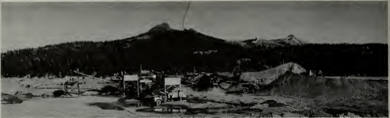
Photo 31. Sand and gravel plant of Tahoe Western Ready-Mix Company at Hope Valley. Camera facing east. Photo by Edmund W. Kiessling.
